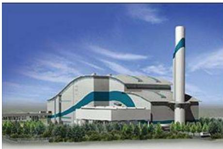
From 2011 the new Von Roll Inova reference plant "Riverside" in the south-east of London will generate 72 MW of electrical energy per year from 585,000 Mg waste.
