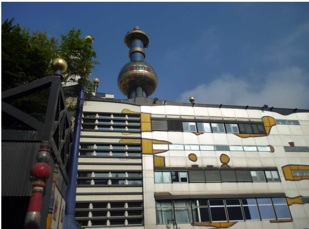
Picture 2. Spittelau, WTE PLANT.
