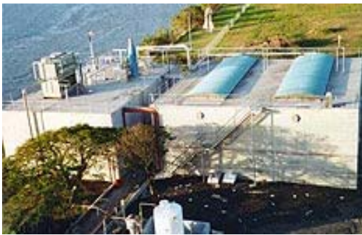
Figure 3, Visy Paper AD Plant, Brisbane, Australia (Field and Sierra, 2003)
