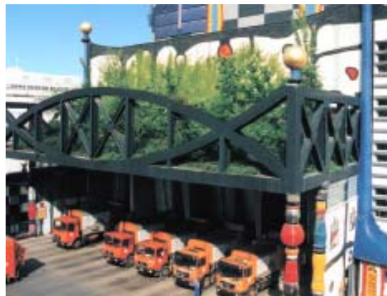
Figure 2: Eight tipping points to unload MSW into the bunker
