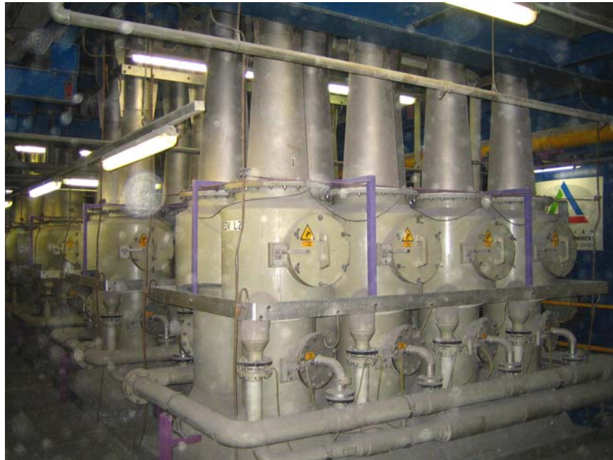
Figure 8: Electrodynamic venturi reduces the dust content to < 1mg/nm 3
