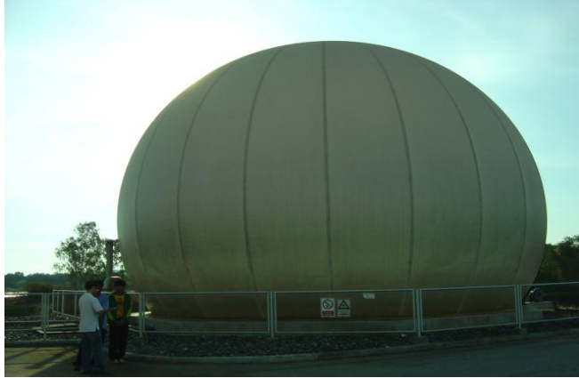
Figure 10: Rayong Municipality 's biogas tank 27
