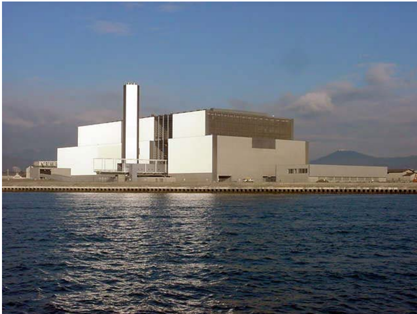
The new Hiroshima WTE uses the Martin grate technology
